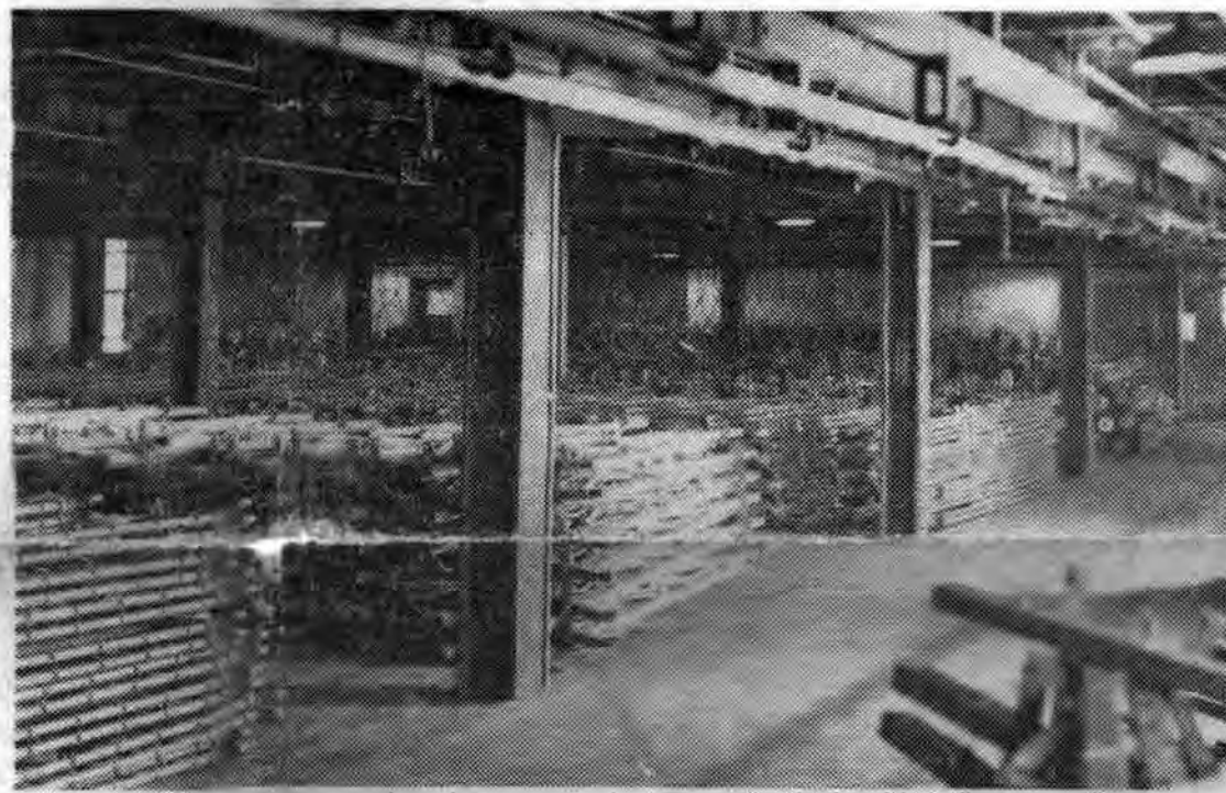
The above photos show the David Bradley warehouses, which are "splitting at the seams!" Everything possible is being done by Management in an attempt to alleviate this condition.
