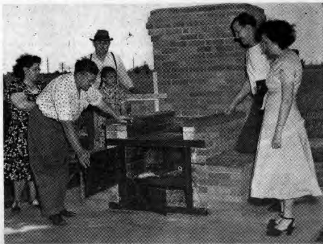
In the foreground is Harry Gilbert (left) of the Experimental Department, examining one of the dutch ovens in the Recreation Park. Mr. Gilbert commented on the beauty and construction of the ovens and said he wouldn't mind having one in his back yard. The others in the picture are (left to right) Mrs. Gilbert, Walter McIntosh and his granddaughter, "Pat" Pattengale and Mrs. Charles Pangle. "Pat" is a pattern maker in the Tool Room.
